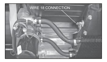
Figure 46. Wire 18 Connection 10-20 kW Units
